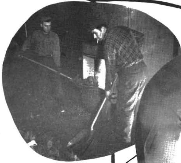
METALS FOR CASTINGS ARE MELTED IN CUPOLA. FIRING CUPOLA ARE TED FOUNTAINE (LEFT) AND JOHN HOLMI. POURING MOLTEN METAL INTO LADLE IS PAUL MENEGUZZO.
