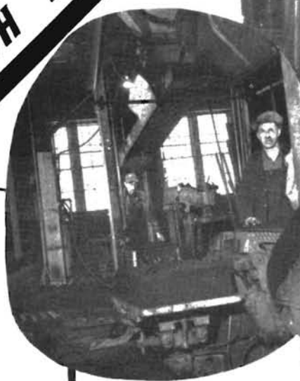
METALS FOR CASTINGS ARE MELTED IN CUPOLA. FIRING CUPOLA ARE TED FOUNTAINE (LEFT) AND JOHN HOLMI. POURING MOLTEN METAL INTO LADLE IS PAUL MENEGUZZO.
