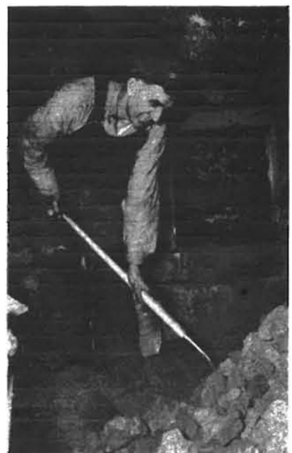
Joseph Primeau, Cupola Charger, shoveling coke into cupola, getting ready for the melt.
