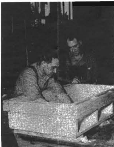
Joseph Harris, pattern maker and John C. Sullivan, helper, making a core box.
